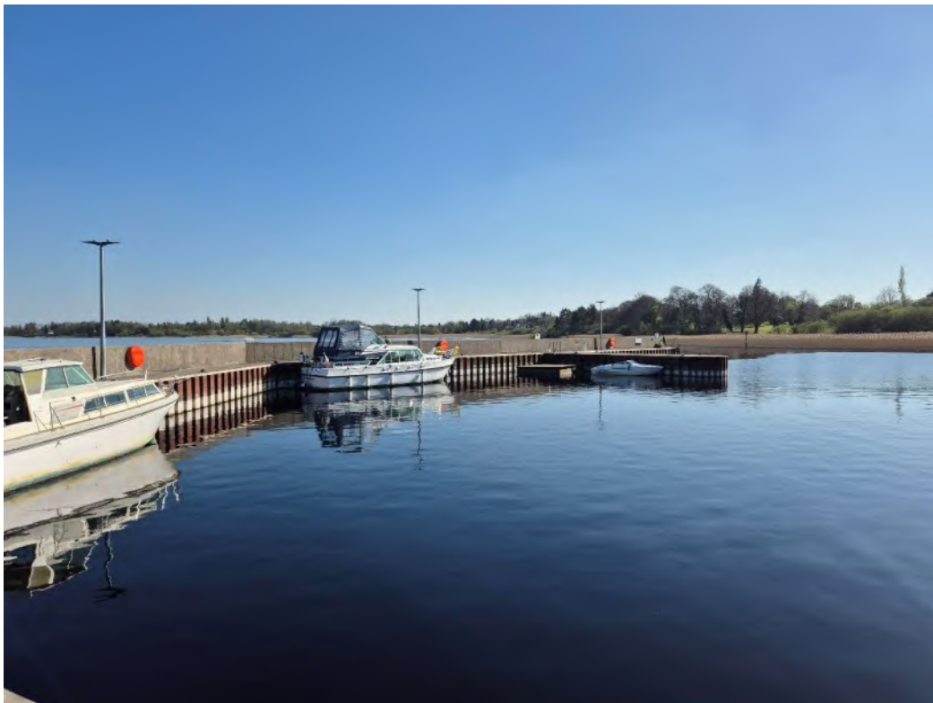
Plate 3-2 The existing Marina at Hodson Bay is a ‘cast-in-situ’ concrete structure.
